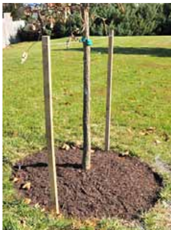
Typical wood staking.
