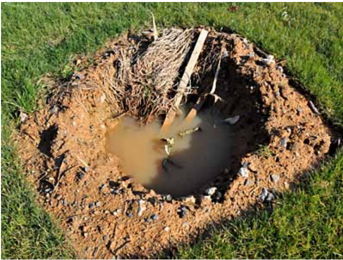
Standing water in planting hole indicates poor drainage.
