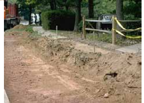
Severed roots due to sidewalk and road construction.
