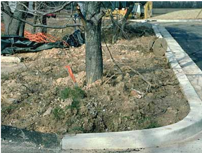
Grade change due to construction.
