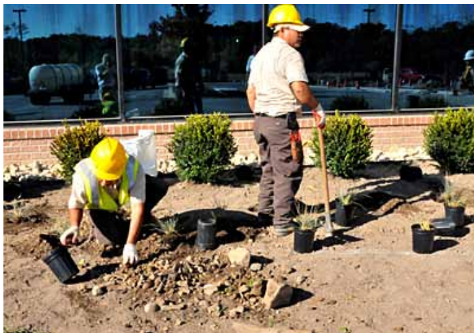
Loosen soil and remove debris before planting.
