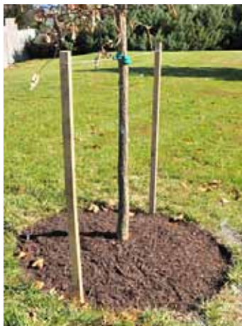
Typical wood staking.
