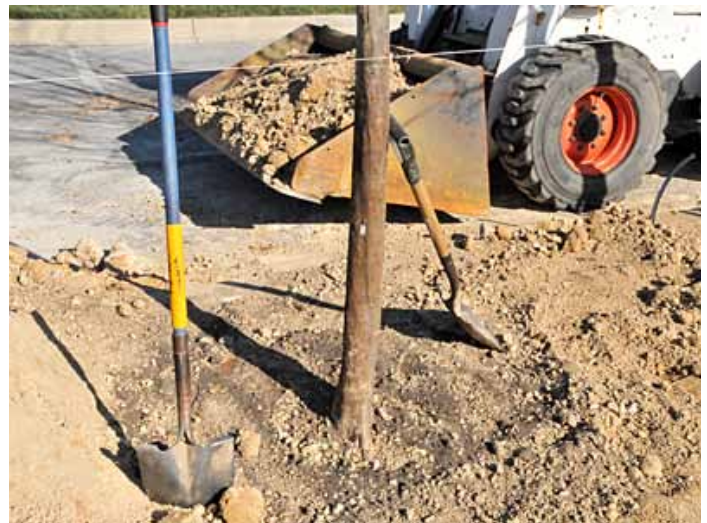
Remove excess soil and properly grade planting area.
