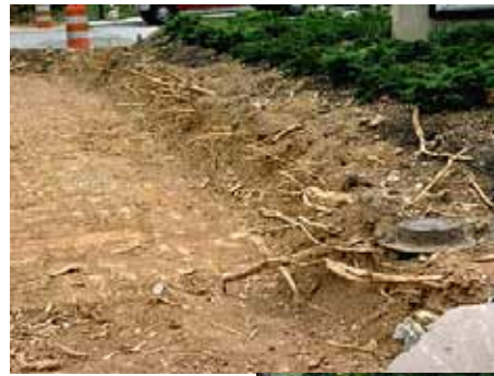
Severed roots due to sidewalk and road construction.
